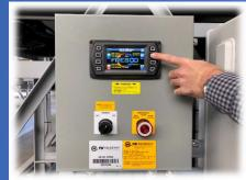
THE PATENT PENDING DESIGN OF THE AERIS COOLING SYSTEM ALLOWS FOR MAXIMUM FLEXIBILITY THAT ALLOWS UP TO FOUR INDIVIDUAL CELLS TO BE OPERATED INDEPENDENTLY IN EITHER AUTOMATIC OR MANUAL MODE THAT CAN RUN **IN ANY COMBINATION OF PARALLEL, SERIES OR SEPARATE PROCESS FLOWS.** EACH CELL IS FITTED WITH 2"NPT CONNECTION TO ALLOW FOR INDIVIDUAL RELIEF VALVE BASED UPON CONDITIONS AND PREFERENCES.
